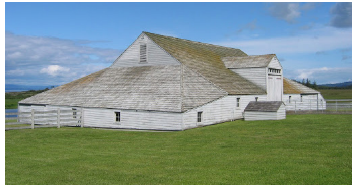
When Peter Lawson announced he was going to build this barn in 1874, he was told the structure would never withstand the winter winds that howl up the Strait of Juan de Fuca. Undaunted, Lawson started work, and a barn-raising was organized by his neighbors. The barn still stands, and the broad axe used to hew the beams is on view at the San Juan Historical Museum. Photo: Tim Dustrude
